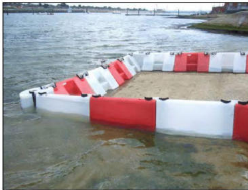
Figure 8 – Typical Self-Weighting Flood Barrier
