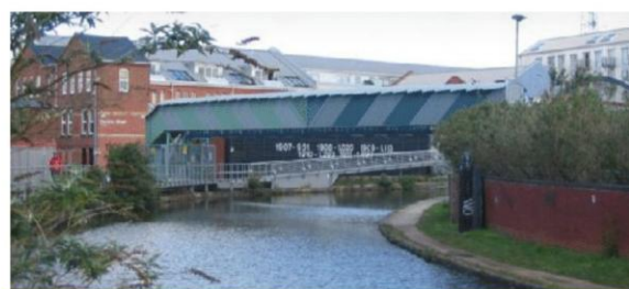
Arden has an extensive canal network that makes a link between the urban and rural areas of this NCA.
